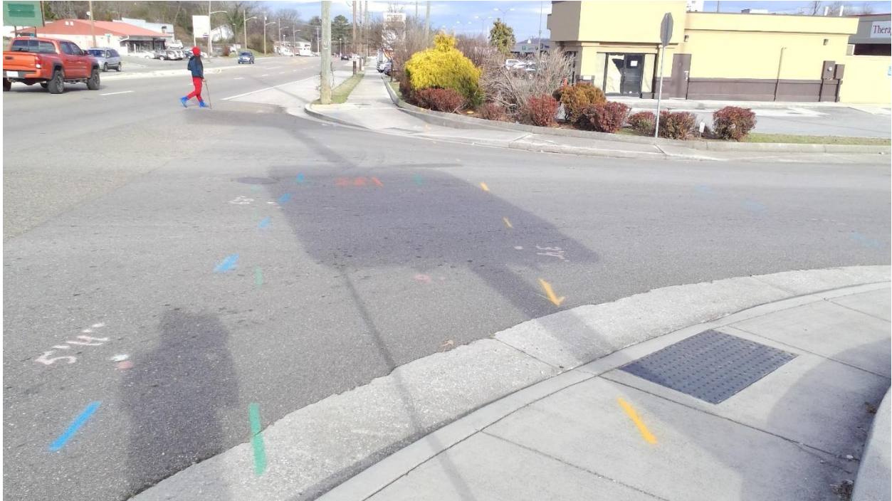
FIGURE 2: ASHEVILLE HIGHWAY (SR 168) AT PARK STREET Demonstrates curb ramps
