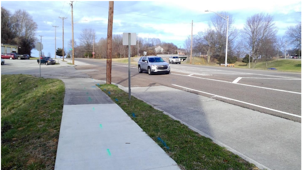
FIGURE 11: RUTLEDGE PIKE (SR 1) Demonstrates curb ramps and sidewalk repairs
