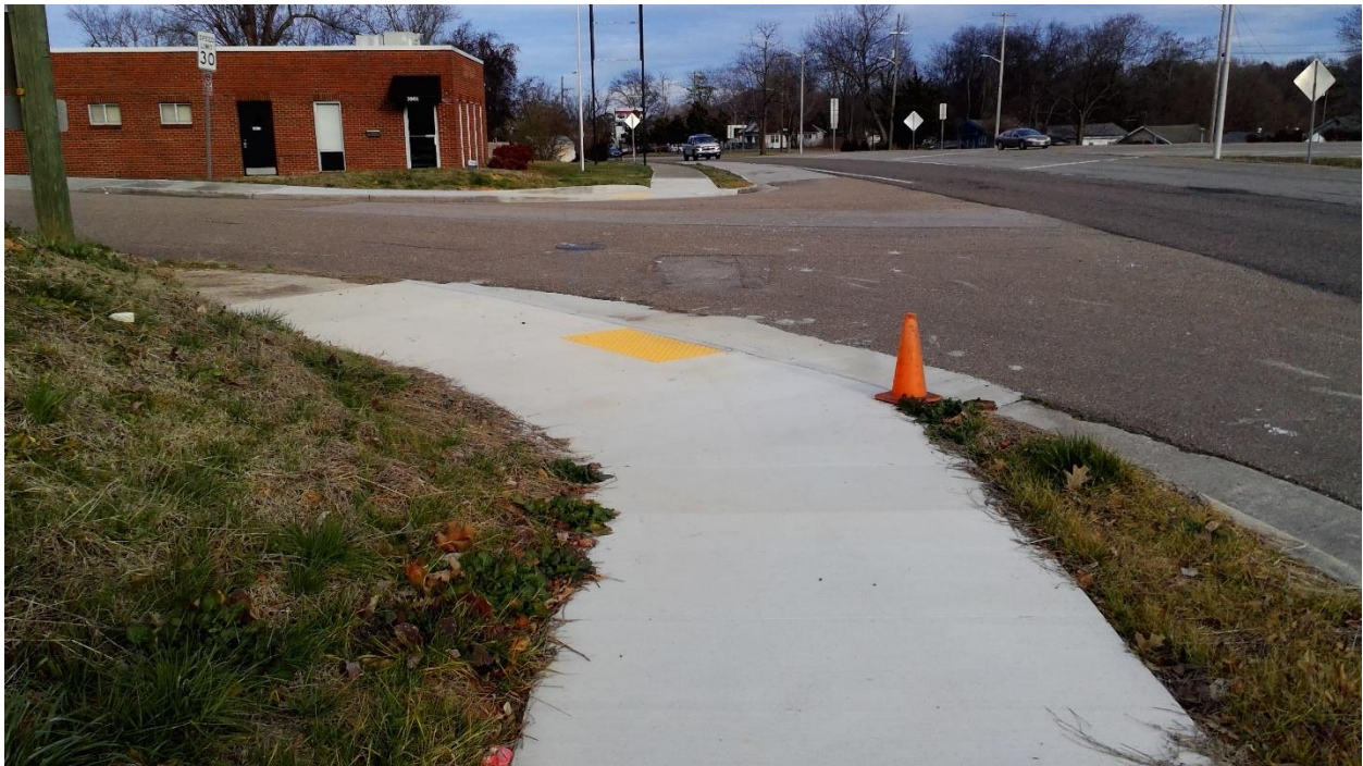
FIGURE 13: RUTLEDGE PIKE (SR 1) AT MCCALLA AVENUE Demonstrates new curb ramps
