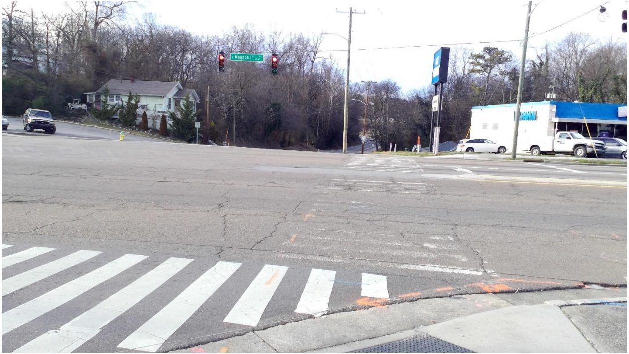
FIGURE 10: MAGNOLIA AVENUE (SR 1) AT PROSSER ROAD Demonstrates no pedestrian signal heads or push buttons, crosswalk markings faded
