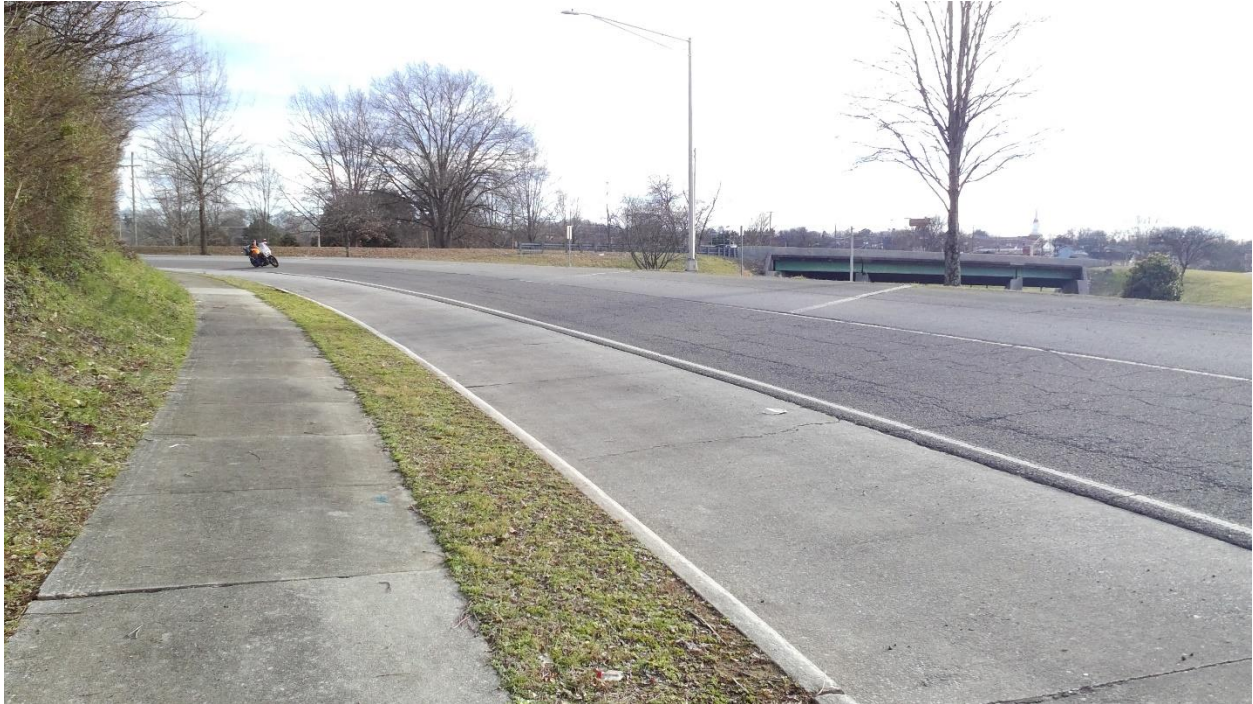
FIGURE 12: RUTLEDGE PIKE (SR 1) Typical sidewalk
